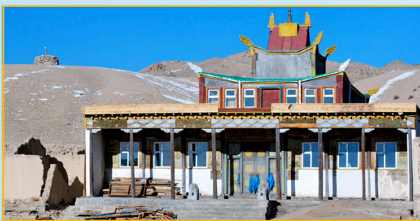
Main temple at Amarbuyant Monastery prior to renovation
